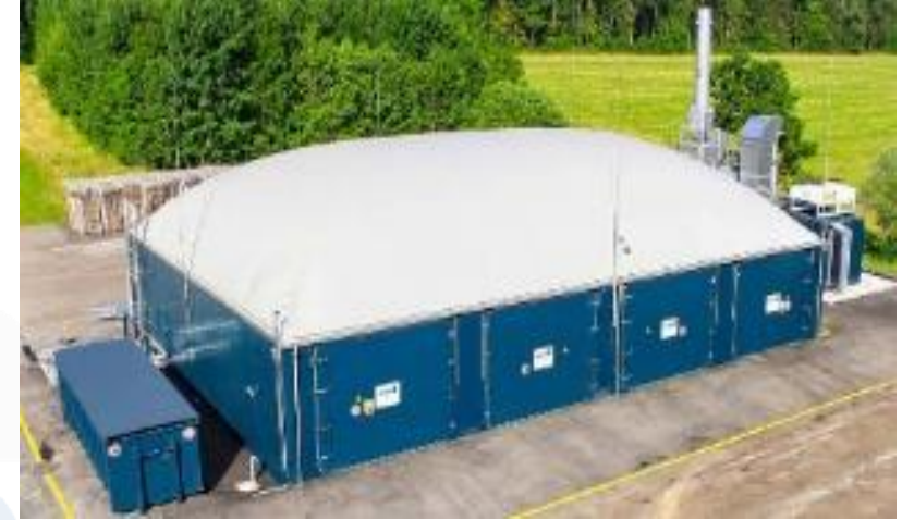
Digester: 1 MW electricity from waste
